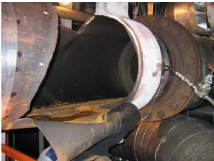
Figure 5. Rupture of nuclear plant feed water pipe, Mihama, Japan, 2004
